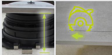
E4. Cut the tile. The dimension of the tile is equal to the distance between the BSJ profile and the SUPACLPP base clip.
