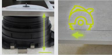
D4. Cut the tile. The dimension of the tile is equal to the distance between the BSJ profile and the SUPACLPP base clip.
