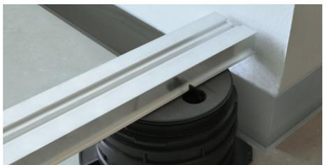
28. Wedge the joist between the SUPA4 tabs of the wall perimeter corner pedestals.
