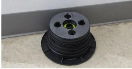
9. Assemble the pedestal and position it with the cut side towards the wall.
