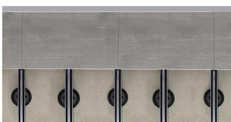
39. Position the first row of tiles perpendicular to the direction of the joists.
