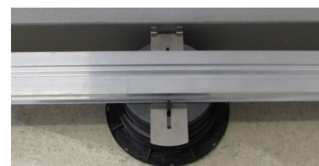
8. Wedge the joist between the SUPA4 tabs of the perimeter pedestals.
