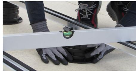
36. Check to make sure that the installation is leveled. If it is not leveled, adjust the height of the pedestals.
