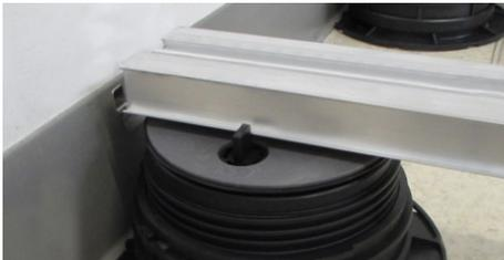
12. Wedge the joist between the SUPA4 tabs of the wall perimeter pedestals.
