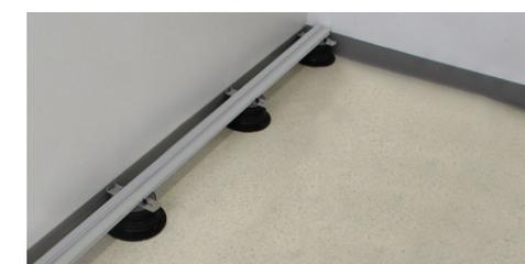
9. Check to make sure that the joists are all wedged firmly to each pedestal.
