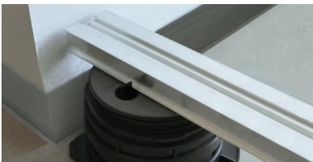
26. Wedge the joist between the SUPA4 tabs of the wall perimeter corner pedestals.
