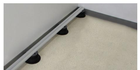
7. Check to make sure that the joists are all wedged firmly to each pedestal.
