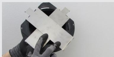
F1. Place two SUPACLPP clips perpendicular to each other under the pedestal base.
