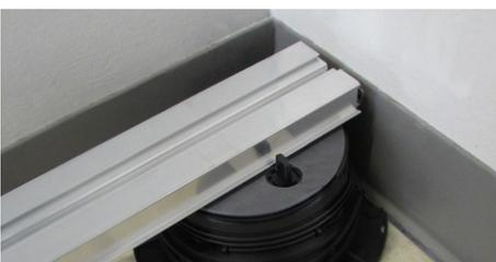
5. Wedge the joist between the SUPA4 tabs of the corner pedestals.
