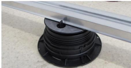
13. Wedge the joist between the SUPA44 tabs of the central pedestals.
