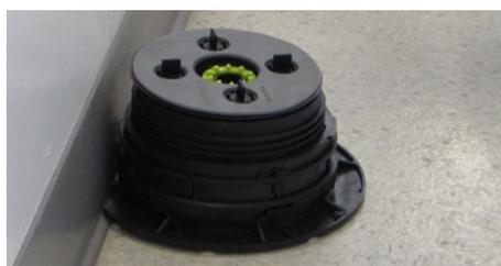
5. Assemble the pedestal and position it with the cut side towards the wall.
