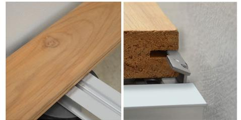
19. Install the first row of wood boards, inserting the groove into the SUPCLIP clip.
