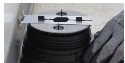
6. Insert a SUPACLPP spacer clip between the two tabs perpendicular to the wall.
