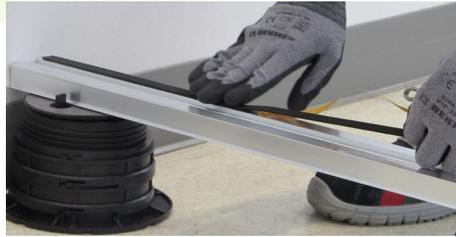
33. Remove the underlying film and adhere the adhesive rubber.
