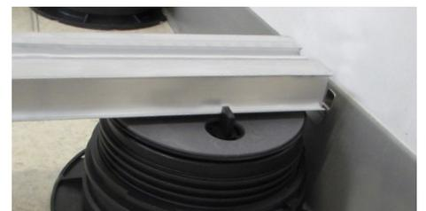
17. Wedge the joist between the SUPA4 tabs of the wall perimeter pedestals.
