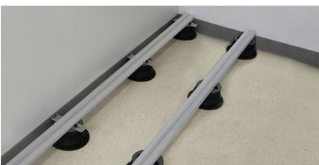
29. Check to make sure that the joists are all wedged firmly to each pedestal.
