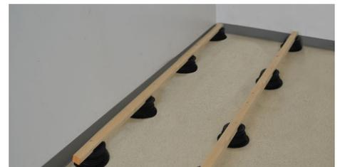
14. Check to make sure that the wood joists are firmly attached to each pedestal.
