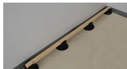
7. Check to make sure that the wood joists are firmly attached to each pedestal.
