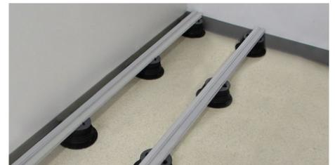
14. Check to make sure that the joists are all wedged firmly to each pedestal.
