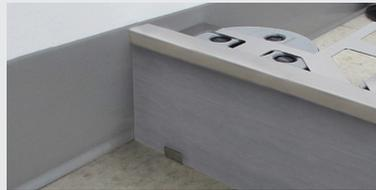
D5. Wedge the cut tile between the BSJ profile and the SUPACLPP clip.
