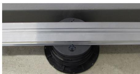
6. Wedge the joist between the SUPA4 tabs of the perimeter pedestals.
