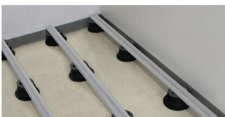
15. Finish installing all joists.
