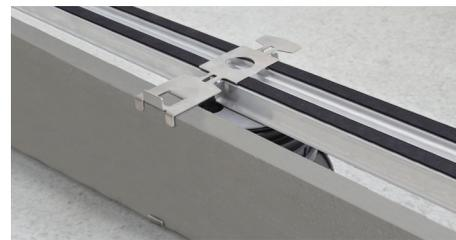
38. Wedge the cut tile between the SUPACLPT clip and the SUPACLPB clip.
