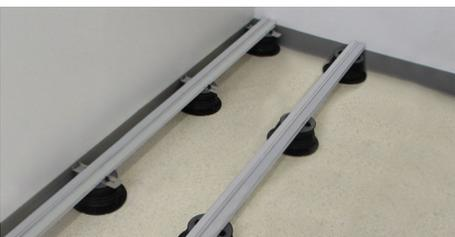
18. Check to make sure that the joists are all wedged firmly to each pedestal.
