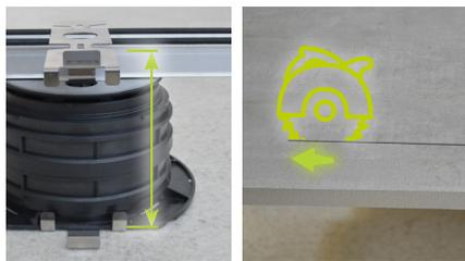
37. Cut the tile. The dimension of the tile is equal to the distance between the SUPACLPT clip and the SUPACLPB clip.
