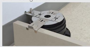
D5. Wedge the cut tile between the SUPACLPT clip and the SUPACLPB clip.
