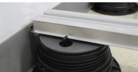
15. Wedge the joist between the SUPA4 tabs of the wall perimeter pedestals.
