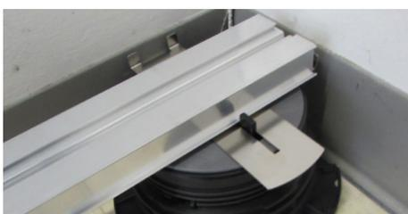
7. Wedge the joist between the SUPA4 tabs of the corner pedestal.
