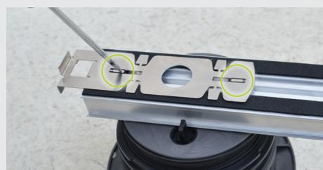
2. Fit the clip to the joist by bending the tabs downwards with the help of a screwdriver.
