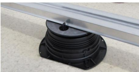
27. Wedge the joist between the SUPA44 tabs of the perimeter pedestals.
