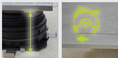
F4. Cut the tile. The dimension of the tile is equal to the distance between the BSJ profile and the SUPACLPP base clip.
