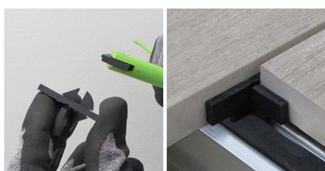
40. Insert the SUPD spacers (removing unnecessary tabs) into the slot on the joist where the staggered tile of the next row will be installed.
