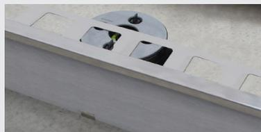
E5. Wedge the cut tile between the BSJ profile and the SUPACLPP clip.
